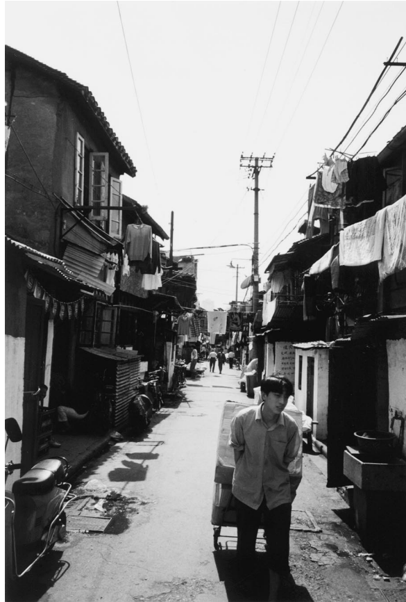
Figure 3 Delapidated housing in the central city of Shanghai
